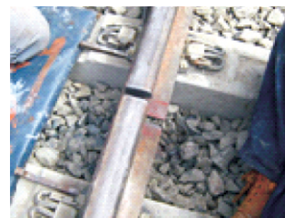
Figure 8.15: Gaps are left in railway tracks to compensate thermal expansion during hot season.
