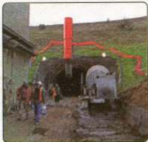
Adit Tunnel Mining
