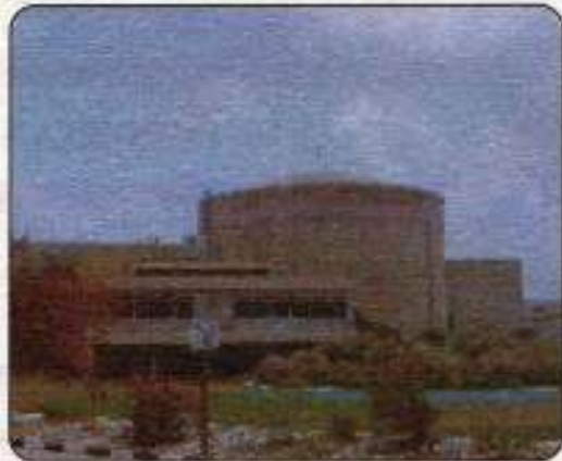
A view of Karachi Nuclear Power Plant
